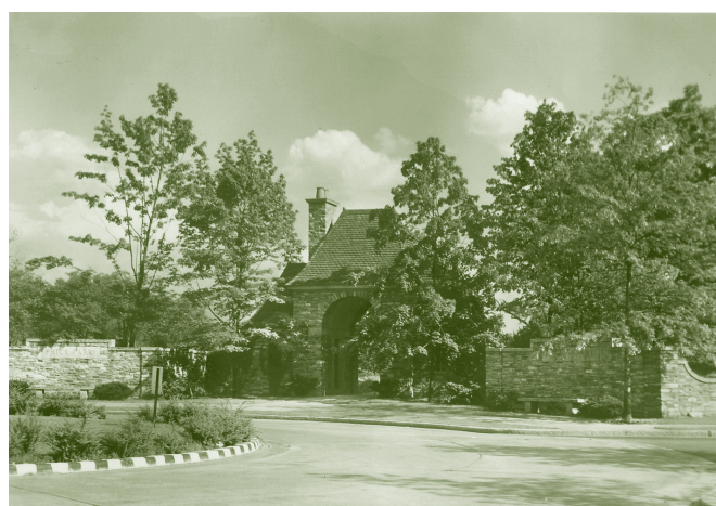
(top) Frick Park gatehouse at Reynolds Street, designed by Innocenti and Webel and restored by the Pittsburgh Parks Conservancy in 2000; (bottom) Historic view of the Frick Park gatehouse at Reynolds Street, designed by Innocenti and Webel, undated photo
