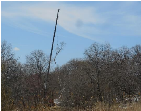
View from Boston side of Riverway Park of tree removal
