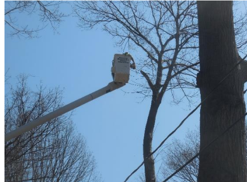
Tree removal in MBTA right-of-way on Carlton Path
