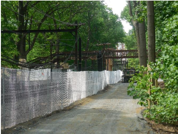
Temporary roadway along MBTA track will allow for heavy equipment
