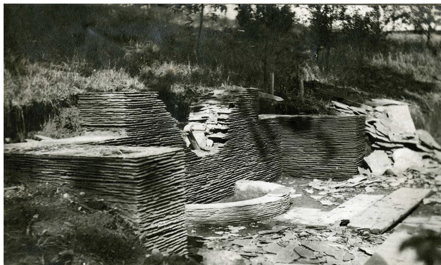
Above left, the 1913 Olmsted blueprint for the Lily Pond—note the backdrop landscape design of shrubs and trees at top and bottom; right, the wall behind the Lily Pond, from which spring water emanates, with its original facing of stacked slate. The slate was replaced in the 1930s with fieldstone, which is consistent with the general Olmsted family style and more durable.
