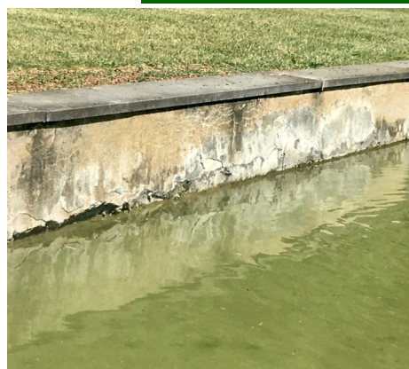
Above, right and center, the condition of the Lily Pond before 2023 reconstruction, including the double east wall at right (note the cracked original 1913 wall on the lower part of the photo); left, an aerial view of the Olmsted-inspired winding path built by the City of Utica to complement this project and enhance the functionality and appeal of the Lily Pond Plateau.
