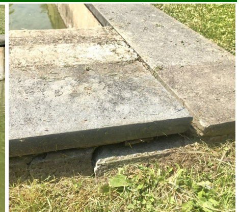
Above, right and center, the condition of the Lily Pond before 2023 reconstruction, including the double east wall at right (note the cracked original 1913 wall on the lower part of the photo); left, an aerial view of the Olmsted-inspired winding path built by the City of Utica to complement this project and enhance the functionality and appeal of the Lily Pond Plateau.
